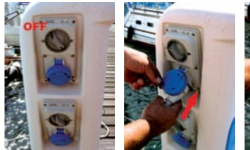
On every electricity pole there are different types of sockets, 16 A (small), 32 A (middle) und 64 - 125 A (large), depending on the electricity power you wish to use. For "smaller" consumers (16 A) the use is very simple, just follow the presented instructions:
